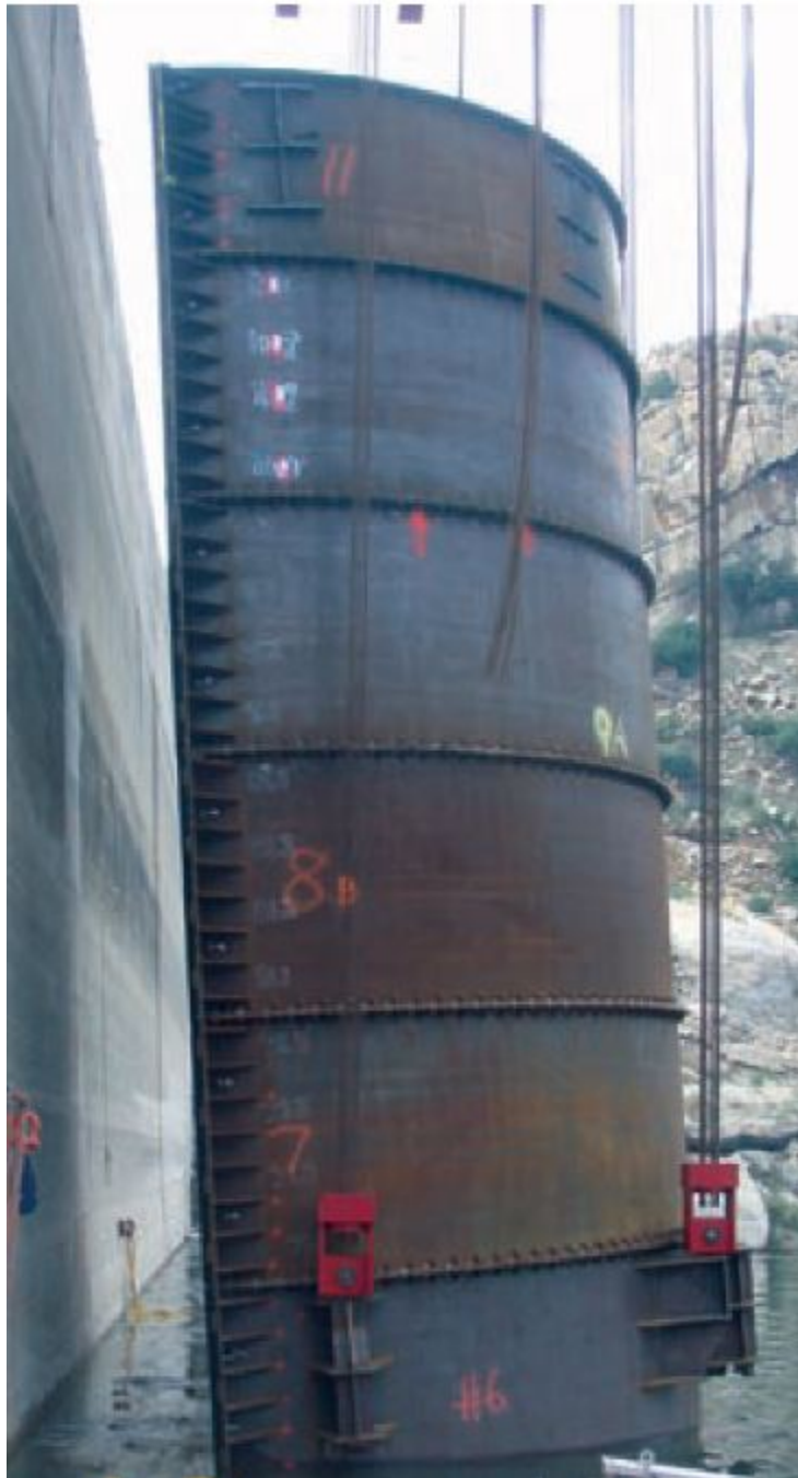
Figure 5-1. San Vicente Cofferdam
