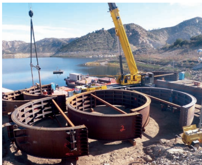
Cofferdam units stored at the edge of the San Vicente Reservoir.
